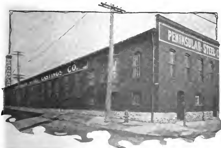
Three-quarter view of the plant of the Peninsular Steel Castings Company, Wight and Iron streets, Detroit, Mich. The company moved into the building shortly after its organization in November
